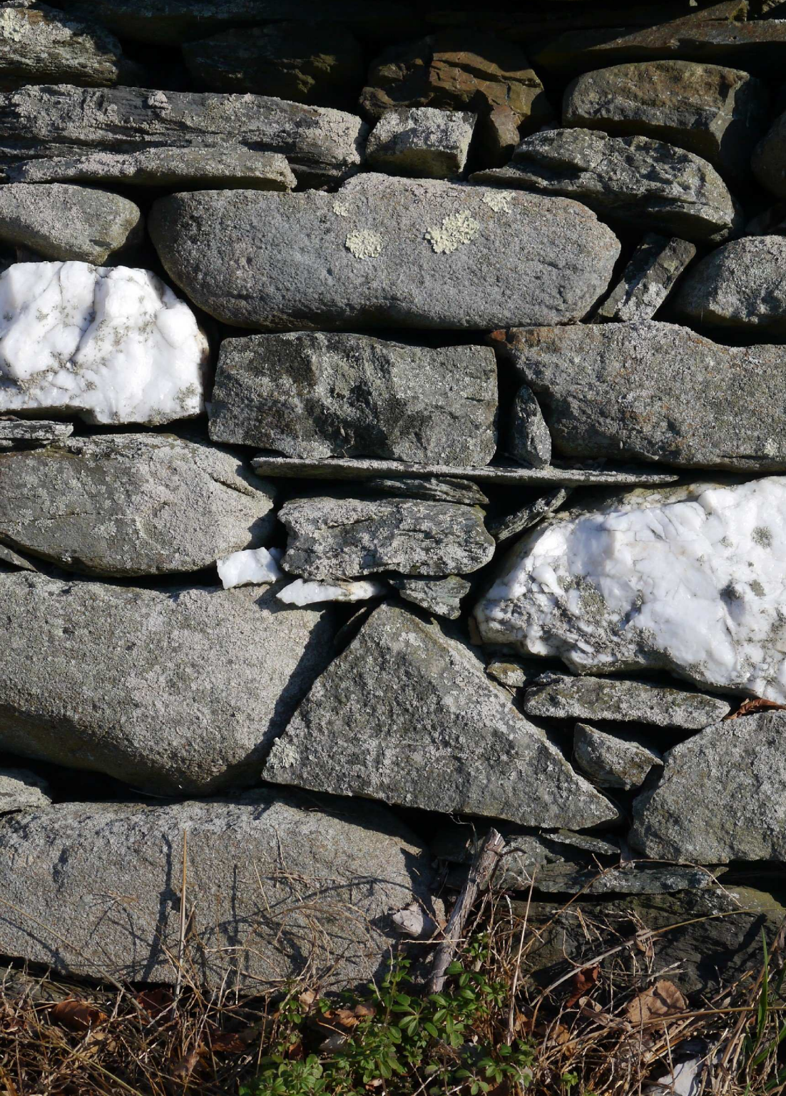
Wall lining Frank Coelho Drive.
